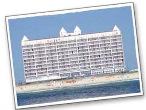
Since installing D-Link wireless products, travellers at the Dunes Manor in Ocean City, Maryland enjoy high speed Internet access in every room.
