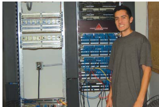
Tornillo Independent School District IT Specialist and Web Designer Carlos Garcia displays D-Link 10GB switches and fiber uplinks.
